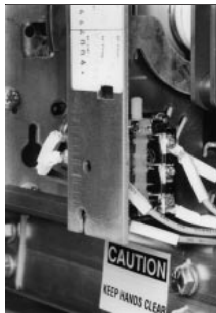
Figure 8: Motor limit switch
